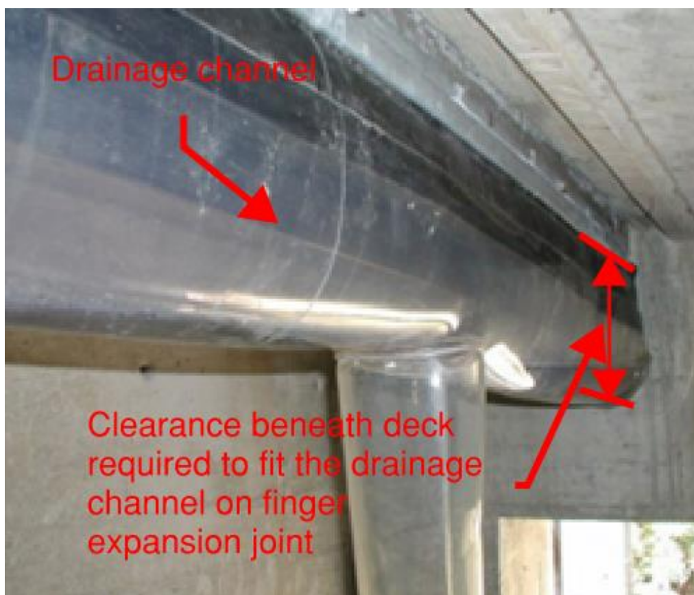
Figure 4: Drainage channel on finger expansion joint [4]
